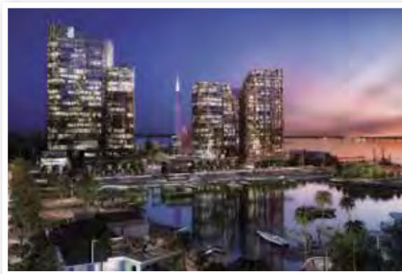
柏斯The Towers at Elizabeth Quay
