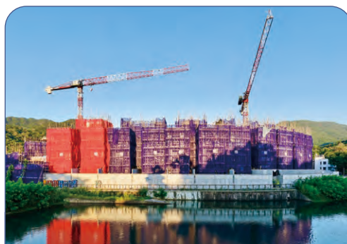
Ho Chung development, Hong Kong
