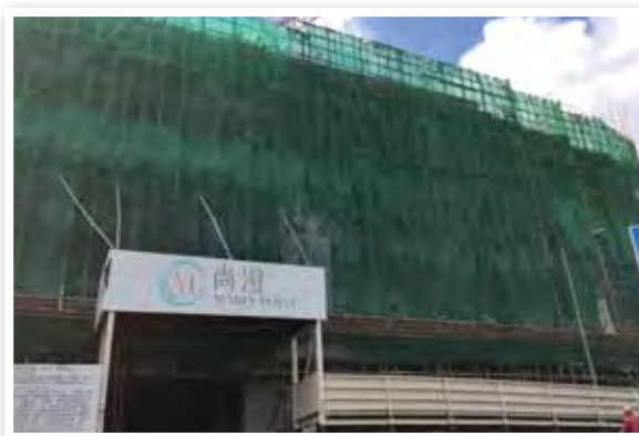
Site of Marin Point, Hong Kong
